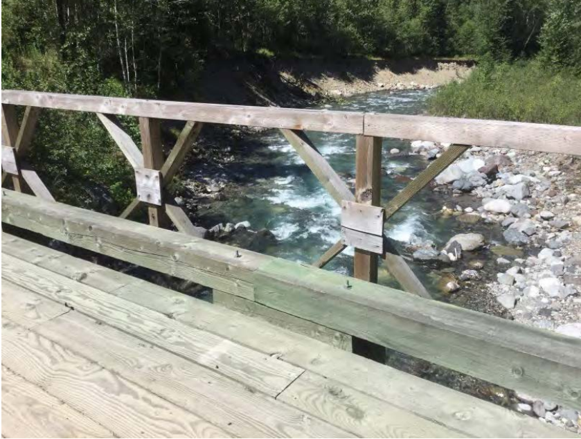
Guardrail and handrail
