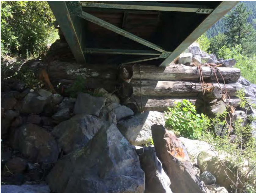
Right Bank Abutment when facing downstream
