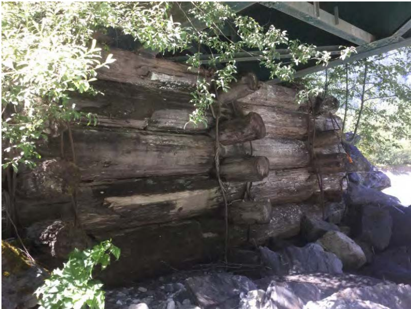
Left Bank Abutment when facing downstream
