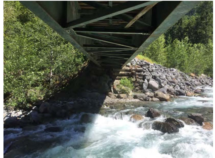
Right Bank Abutment when facing downstream
