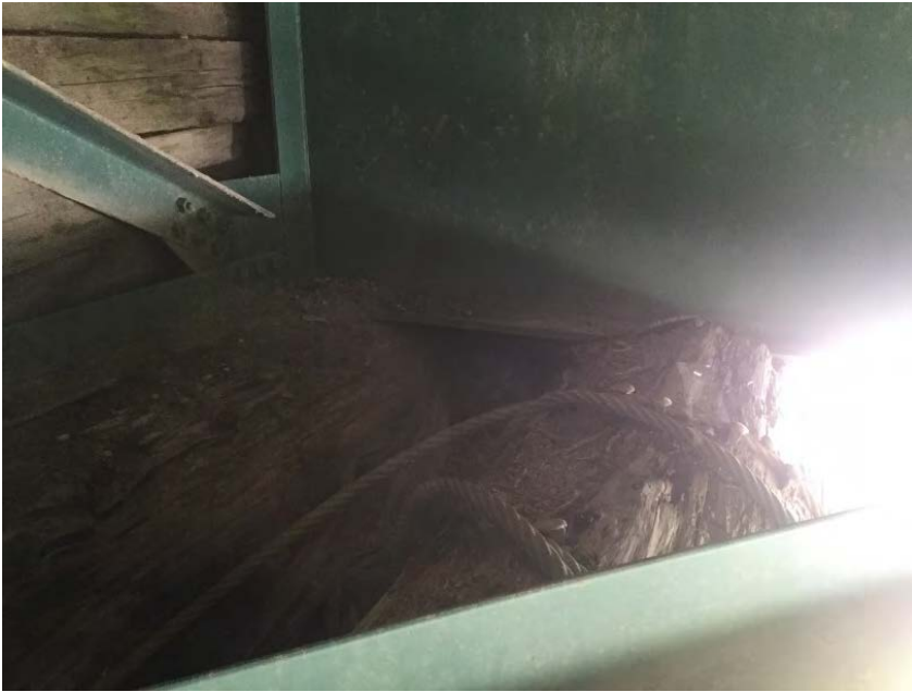
Right bank abutment bearing in 2 locations - both upstream and downstream
