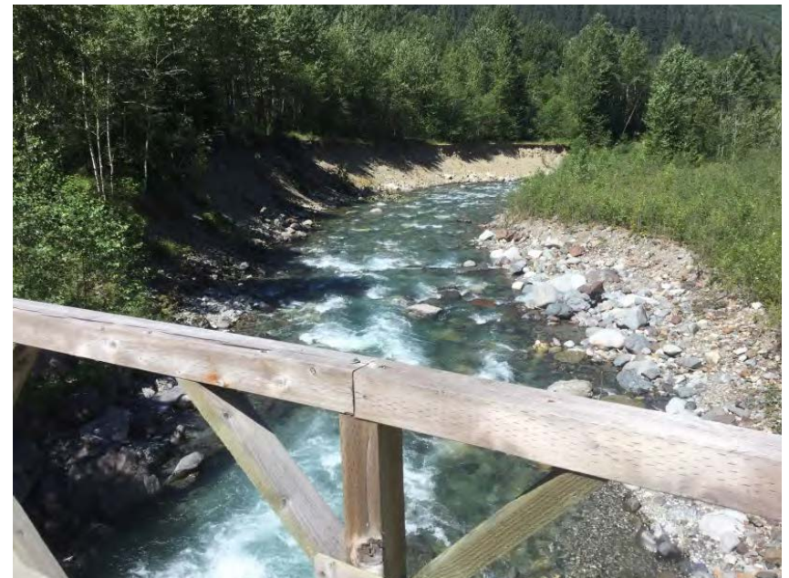
Looking downstream from deck
